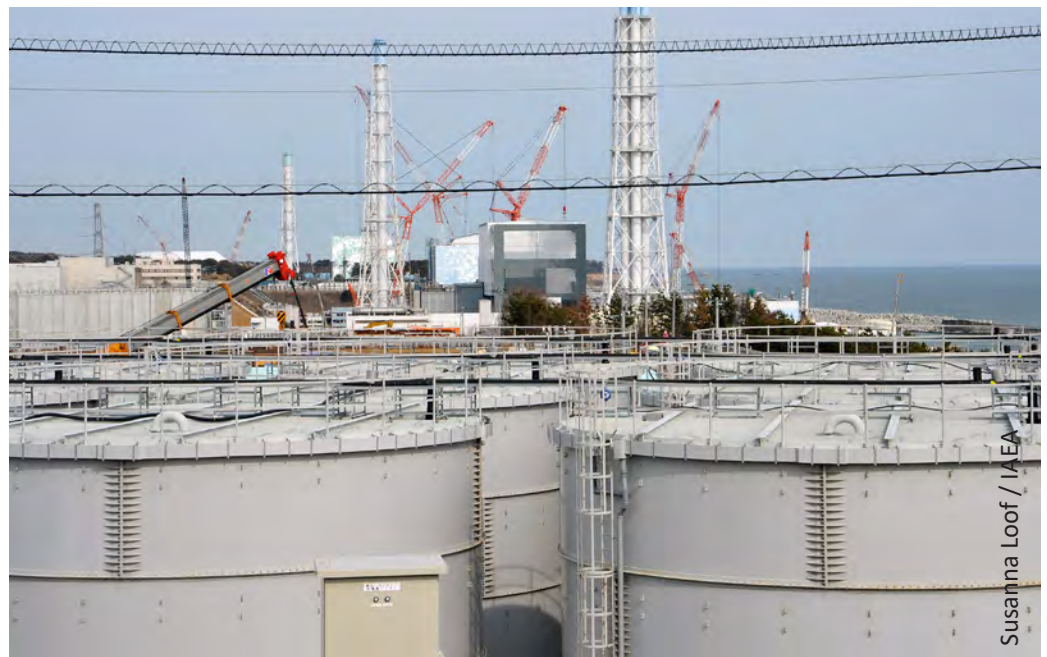
Radioactive water storage tanks
