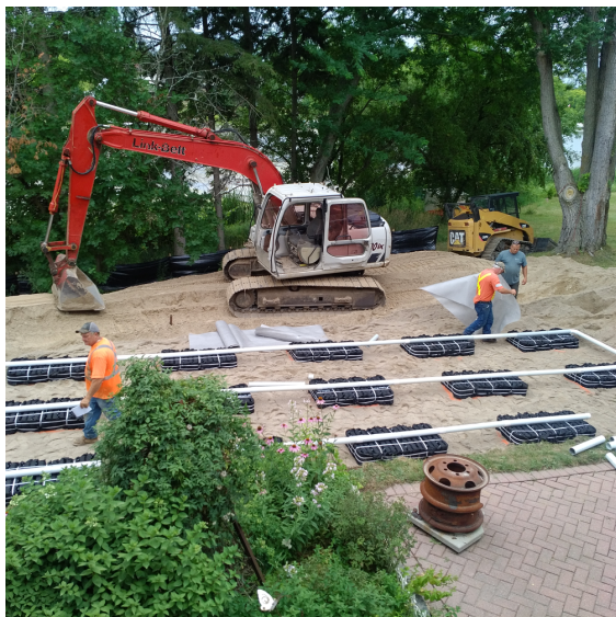
Figure 2. New Tertiary Septic System Installment Following a Failed Inspection of the Previous System [Photo Credit: Liz Huff]
