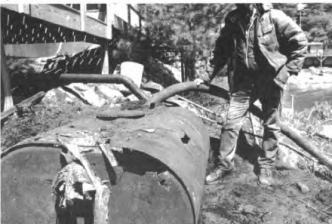
Detritated sewage disposal systems like this are common along the St. Lawrence River.
