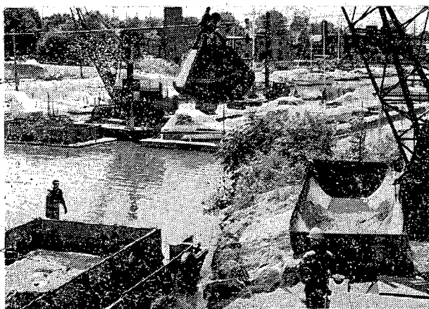
Dredging of contaminated sediment from Trail Creek (Credit: Tom Anderson)
