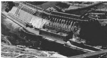
As part of its efforts to meet surging demand for electricity, Ontario Hydro plans to expand its Sir Adam Beck Generating Station on the Niagara River.
