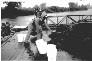
US Army Corps dredging Buffalo River contaminated sediments for testing in ARCS program.
