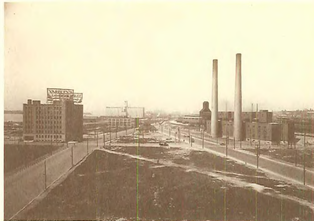
The same view in 1930, showing the graded fill and buildings that have replaced the waters of Toronto Bay. Toronto Harbour Commission Archives, PC 111/9417.
