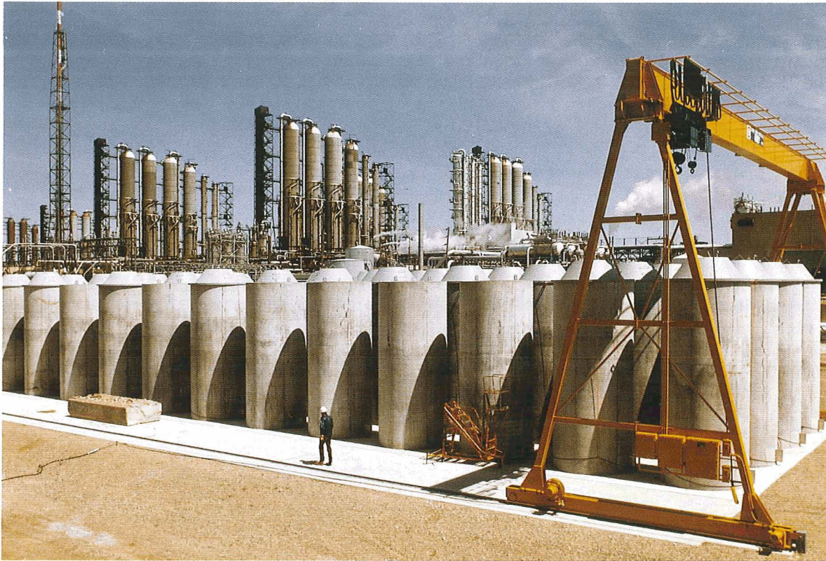
FIGURE 2-8: Dry Storage Canisters at the Douglas Point Reactor Site in Ontario
