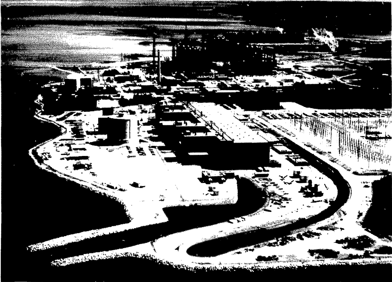
Figure 6 Bruce Nuclear Power Development, from Lake Huron. Bruce B is in the foreground, with the vacuum building very prominent. The heavy-water extraction plant is directly beyond, with the Douglas Point reactor (now being decommissioned) on the left. Bruce A is visible in the far background.
